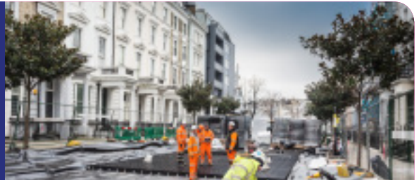
Permavoid installed at Kensington Park Terrace, London
